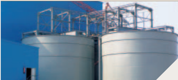
Leach tanks with tank top structure
